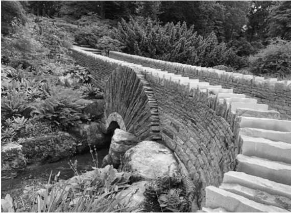
New (dry stone) bridge at Harlow Carr. Looks amazing
